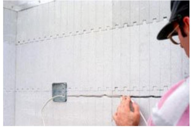
Utilities are typically recessed into cutouts in foam after concrete has been
