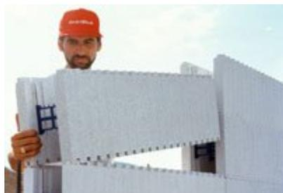
*Stacking preassembled ICF formwork*
